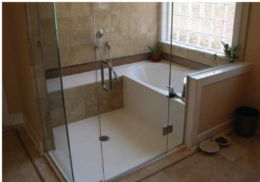
Water Ways: Shower stalls and seats are safer and easier to use than bathtubs, which is why many homes with universal design features incorporate them.
